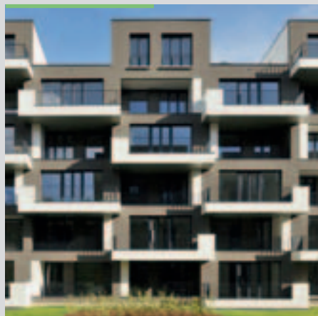
BALCONY APARTMENTS SLOVINSKO
