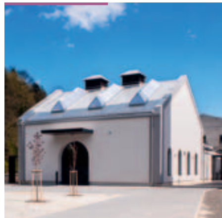
FORMER BOILER HOUSE ČESKÁ REPUBLIKA
