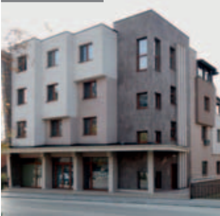
RESIDENTIAL BUILDING "TRAKIA IMPEX" BULHARSKO
