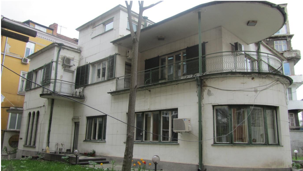
Pictures before ADMINISTRATIVE BUILDING on RLL IX-5,6,14, grid 547, SOFIA, 25A Tsar Osvoboditel Blvd.
